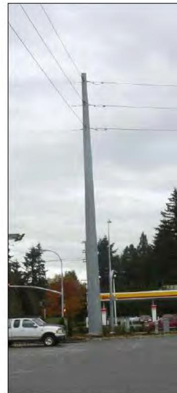
Single-circuit 115 kV steel pole
