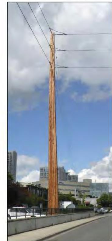
Single-circuit 115 kV glu lam pole
