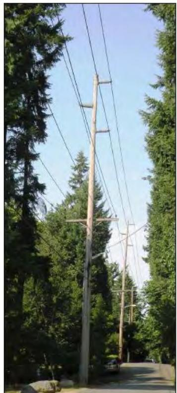
Single-circuit 115 kV wood pole with distribution underbuild
