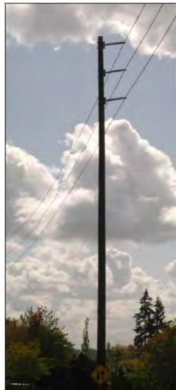
Single-circuit 115 kV wood pole with insulators on one side
